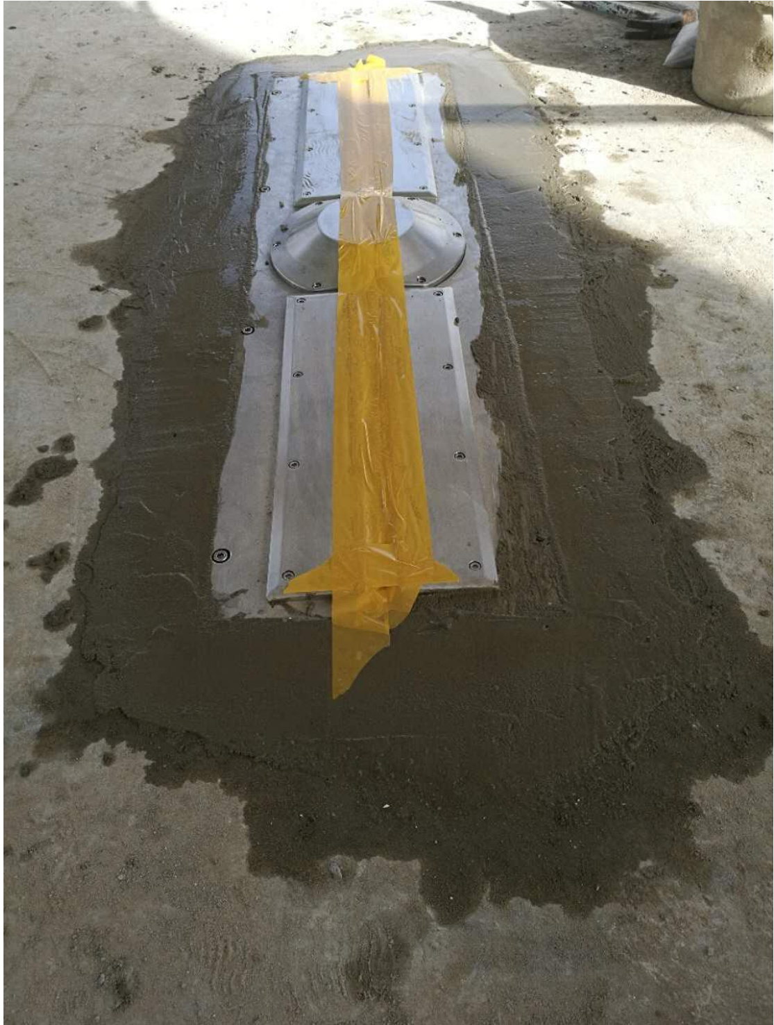
After the installation has been completed
